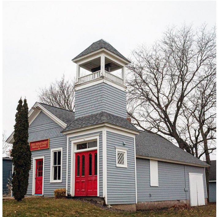
The Firehouse/City Hall after renovation.
