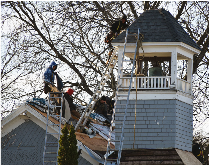
ABC roofing employees at work on the Firehouse.
